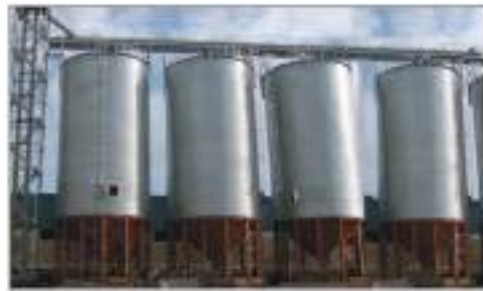
Fig. 5.2.7 Grain storage silos
